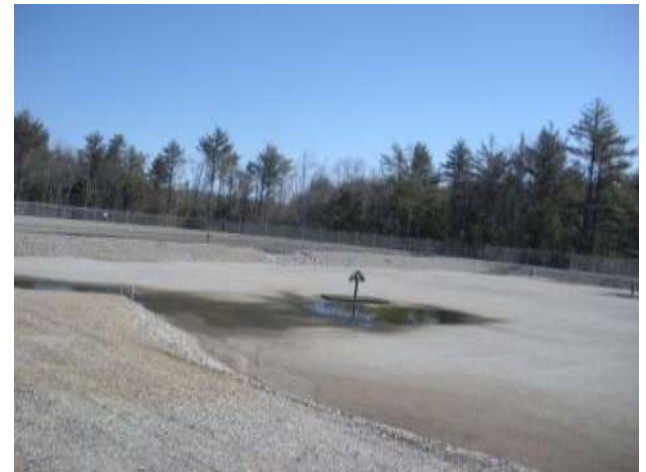
RIB=Rapid Infiltration Beds
