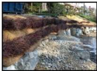
Bio-engineered slope treatment
