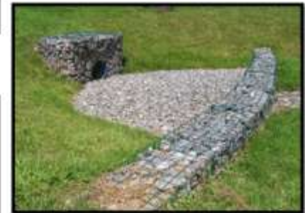
Plunge pool with gabion level spreader
