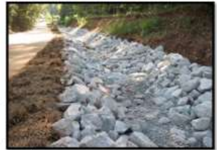
Riprap swale with reinforced shoulder
